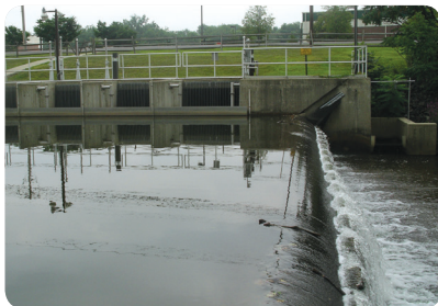
Inflatable Rubber Dam
