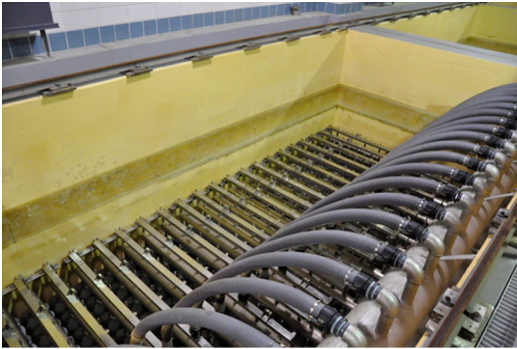
A submerged rack of membrane filtration modules
