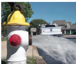
Hydrant flushing
