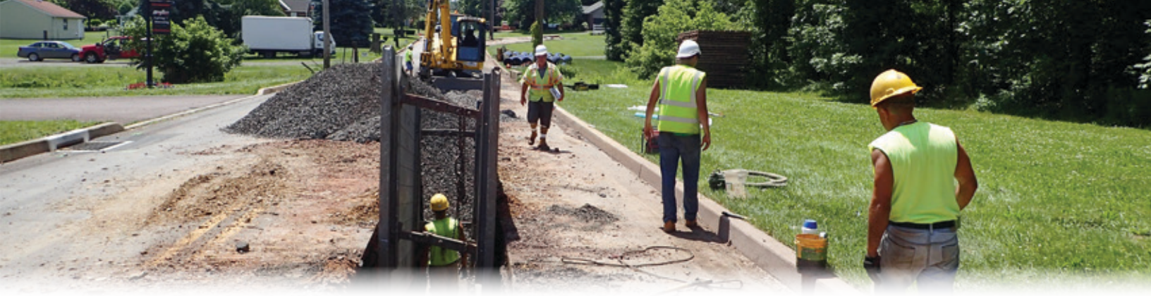
Water Main Replacement work being done on Penn Street in Hatfield.
