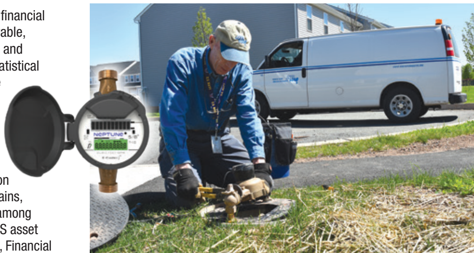
Meter Department Field Service Representative inspecting a water meter in a residential meter pit.
