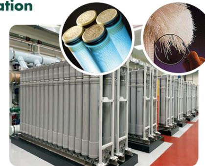
The entire membrane system consists of millions of hollow tube fibers that remove impurities larger than .1 microns, which is smaller than one human blood cell. The surface area of all the membrane fibers combined would cover just over 30 football fields. The filtered water flowing through each fiber flows into a common pipe and is pumped to the next stage. Membrane filtration is one of this plant's most notable features and is considered the filtration technology of the future.
